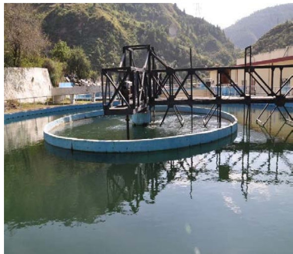
Clarifiers are vulnerable to sloshing and ground movement. Image courtesy SJPNL.
