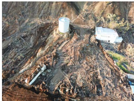
Atsuma Water Purification Plant destroyed by an earthquake-induced landslide in the 2018 Hokkaido Eastern Iwate Japan Earthquake. Images courtesy GEER, 2019.
