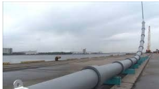
Earthquake resistant ductile iron pipe. Image courtesy Kubota Corporation.
